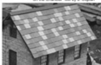
All 4 colors of slate - Red, Grey, Sea Green and Purple were used randomly on the Chandler Mill by J. Coplan
